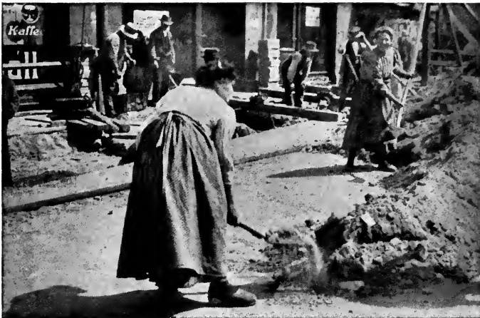
Digging the Tunnel for the New Underground Railway in Berlin.
